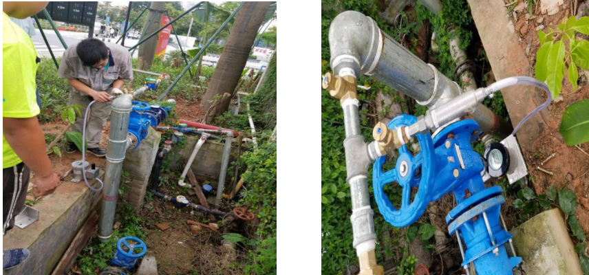
Figure 5. Pressure gauge installation at critical node
