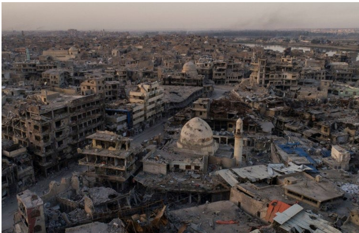
Figure 2. 2: Destroyed buildings and shops in the Old City of Mosul, Iraq. The scope of destruction in the neighborhood is comparable to some of the worst urban battles of World War II. Source: Dana (2017).
