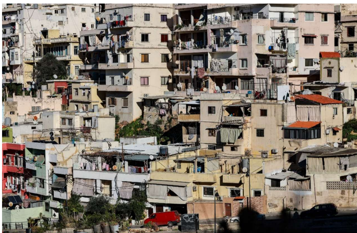
Figure 2. 11: Informal residential urban slums in Tripoli, Lebanon, following the end of that country's 15-year civil war in 1990. Source: Eid (2022).
