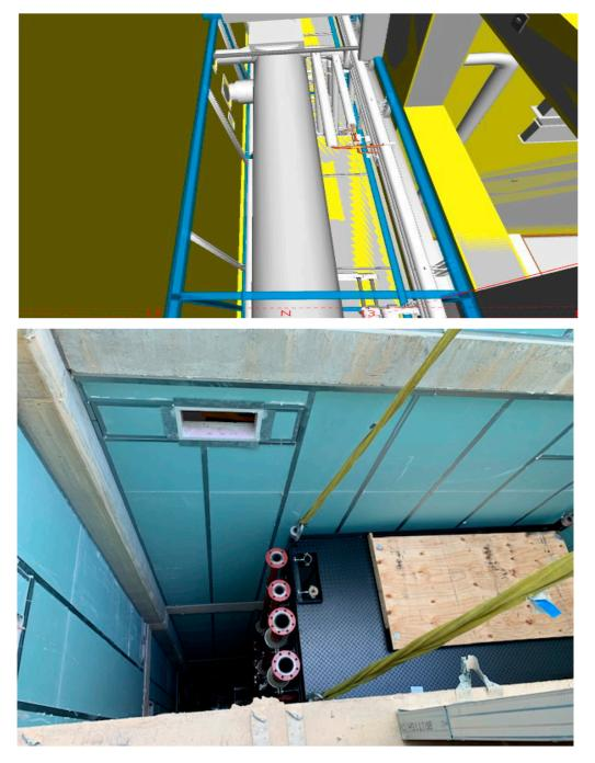
**Figure 4.** Mechanical Riser Module after installation on site (**bottom** image) and how they are represented in a BIM model (**top** image).
