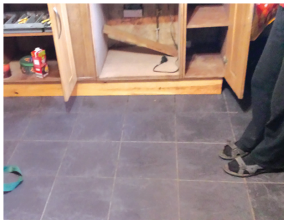
Marine ply kitchen units, with solid oak doors – can be hosed down and disinfected (picture taken 10 days after flood).
