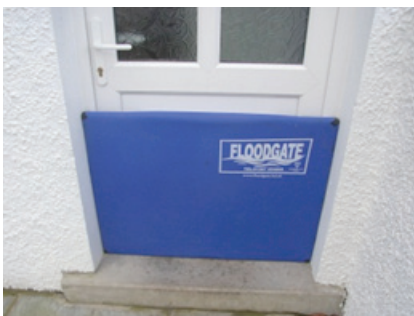
Might not be possible to keep water out entirely but water exclusion / minimisation strategy employed
