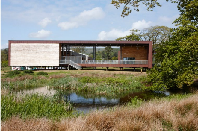
Figure 4 : Margam Discovery Centre frames views through copper clad 'portals'
