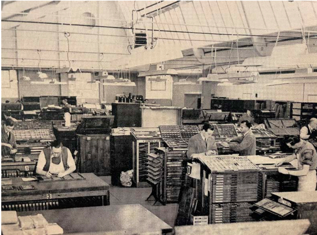
Figure 5.3. The composing department, comprising the 'Oriental', magazine, book, and jobbing sections of the type foundry of Stephen Austin & Sons. From author's personal copy of The story of the opening of the new factory at Caxton Hill , Stephen Austin & Sons, 1954.
