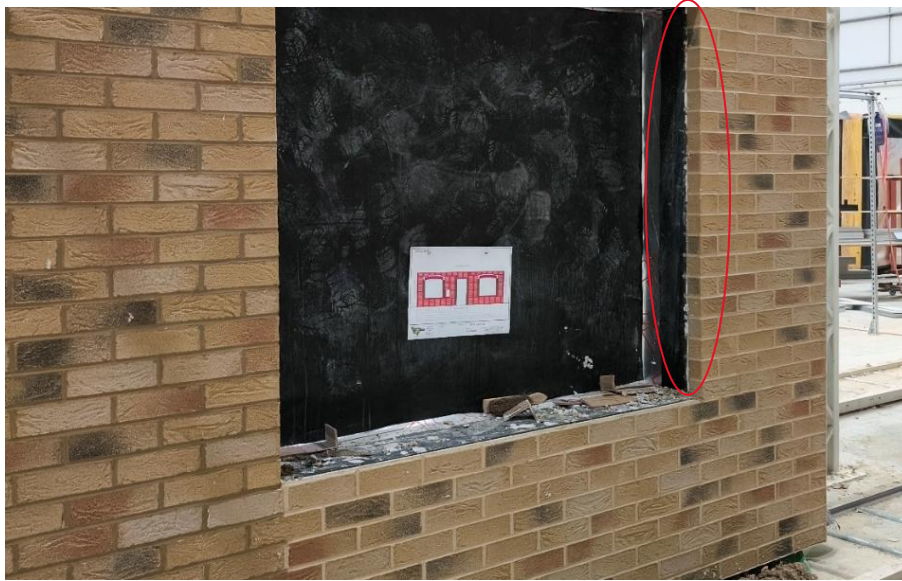
Figure 5.24: Brick slip corner with half brick depth
