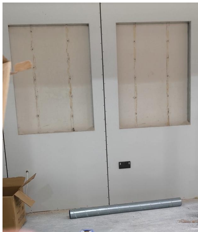
Figure 5.6: Plasterboard opening offcuts
