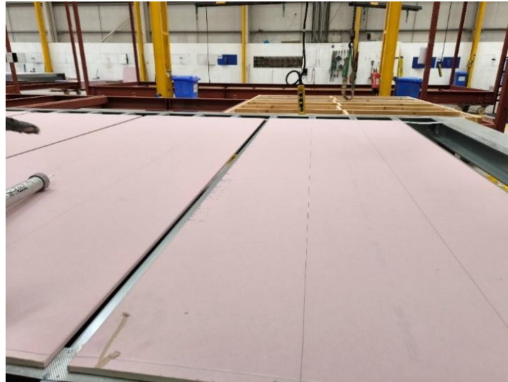
Figure 5.4: Ceiling plasterboard assembly activities
