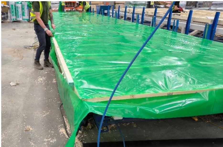
Figure 5.22: Polyethene vapour barrier offcuts
