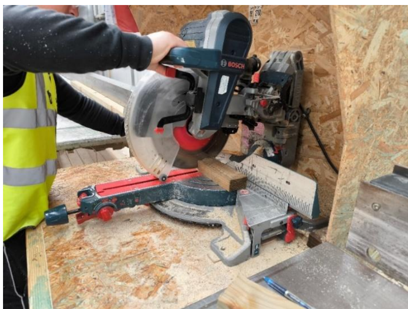
Figure 5.26: Timber battens cutting activity
