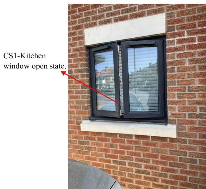
Figure 5. 21: Kitchen window in a partially open position, illustrating occupant ventilation preference during cooking.
