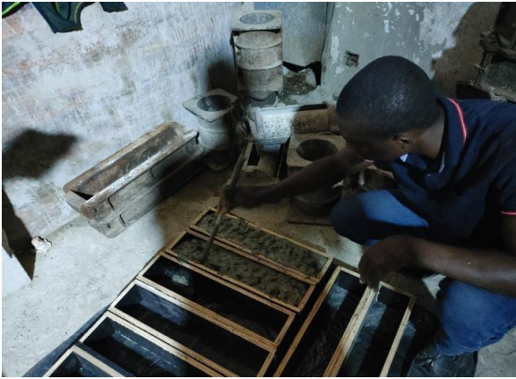
Fig. 3 Casting short column concrete
