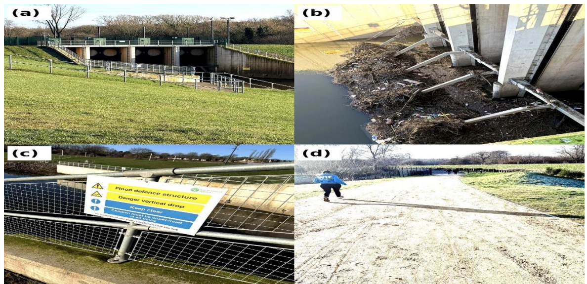
(a) Primary spillway and associated control structures; (b) Debris accumulation at outlet gates during winter conditions; (c) Flood defence safety signage and restricted access; (d) Public use of the circular footpath across the embankment during winter conditions.
