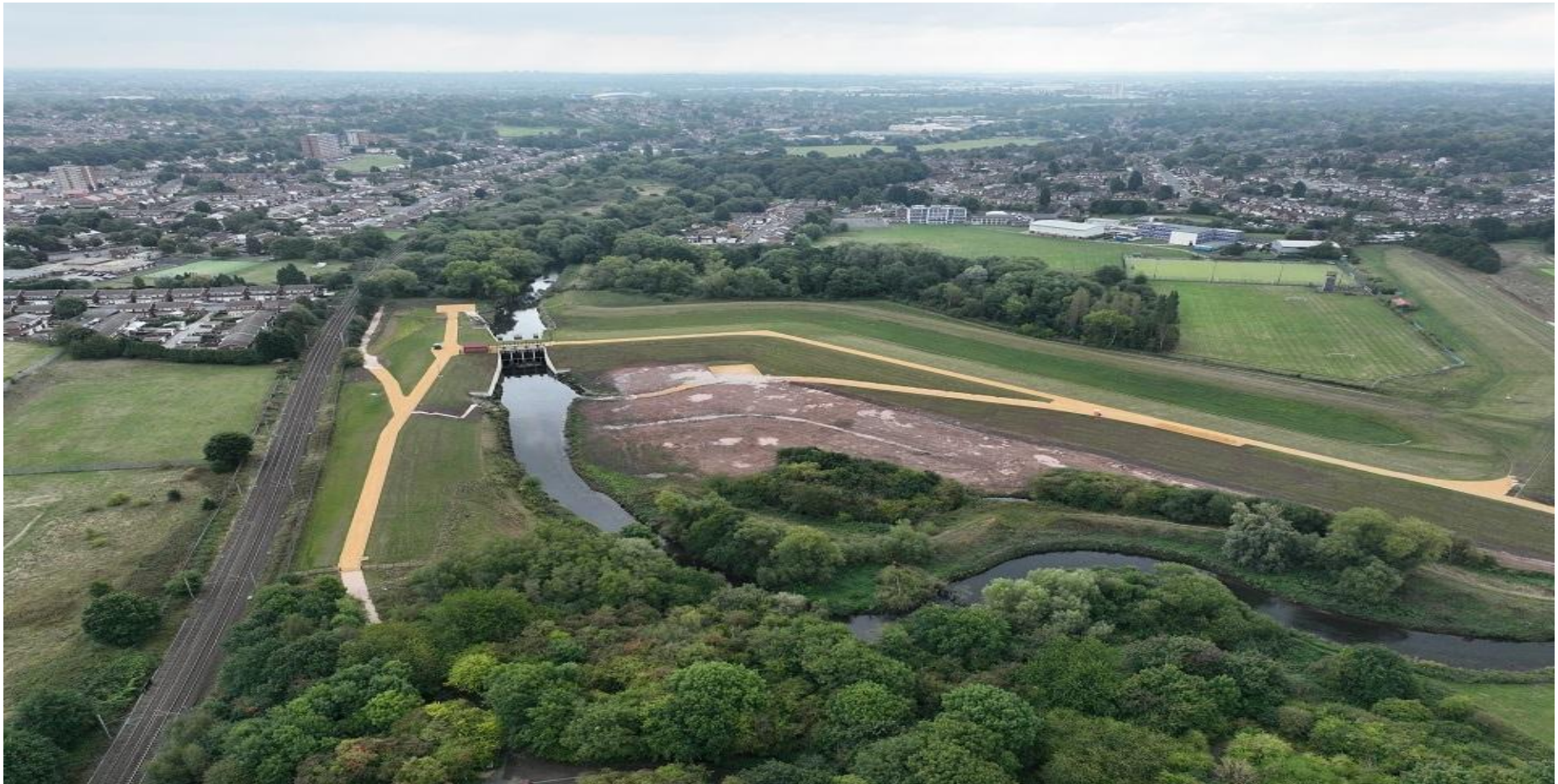
Figure 7.1: Location of the Forge Mill Flood Retention Reservoir (EA, 2023c)
