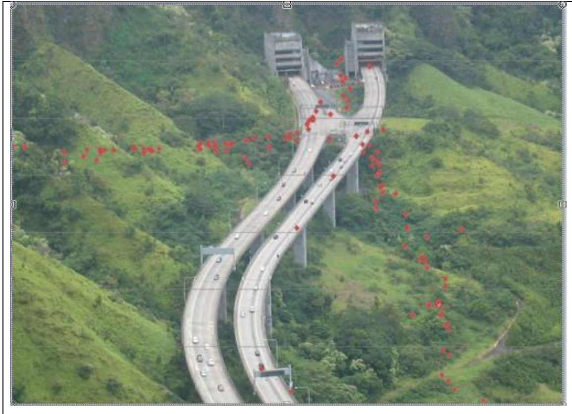
Figure 7.26. Participant did not like ‘hanging motorway made of concrete in the green environment.
