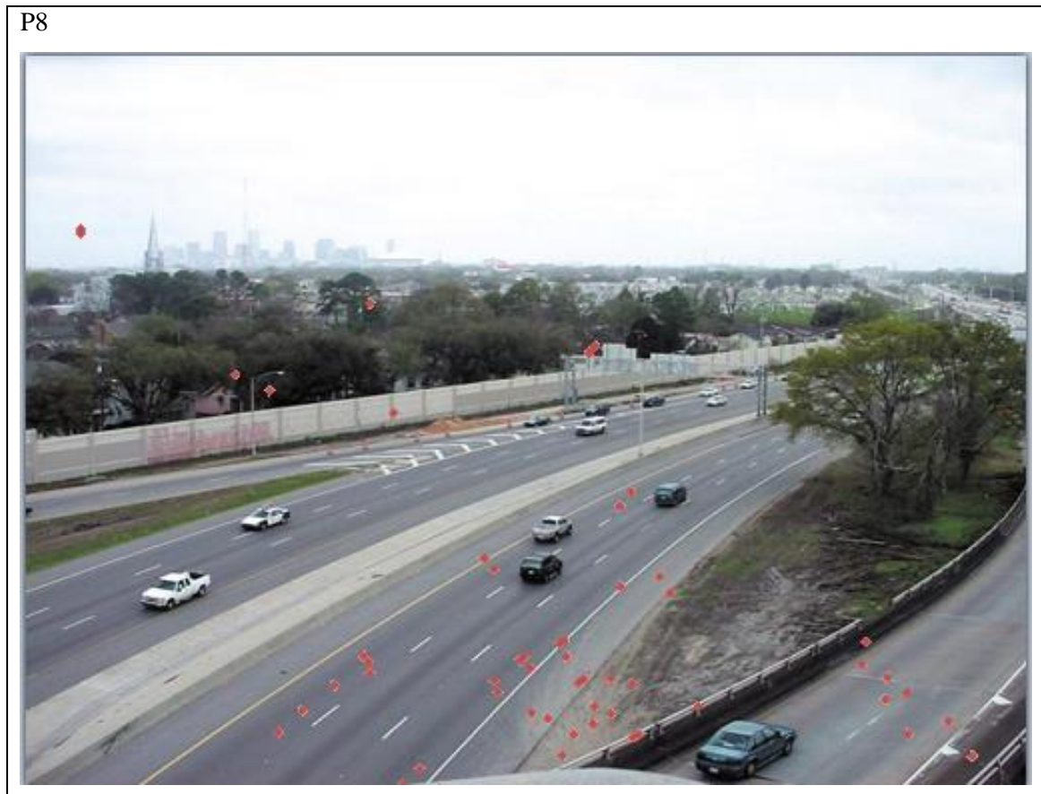
Figure 8.35. Image showing a motorway with many of fixations.
